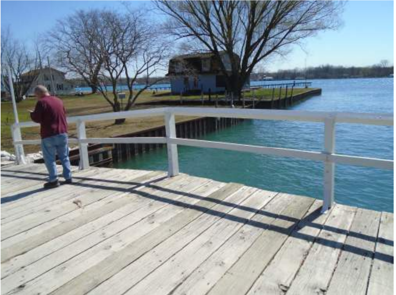
Looking NE at railing and deck
