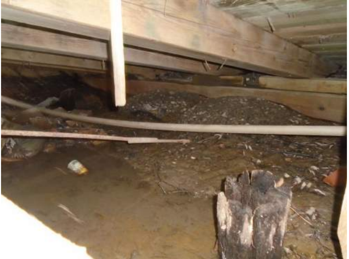
Looking south at south bearing beam
