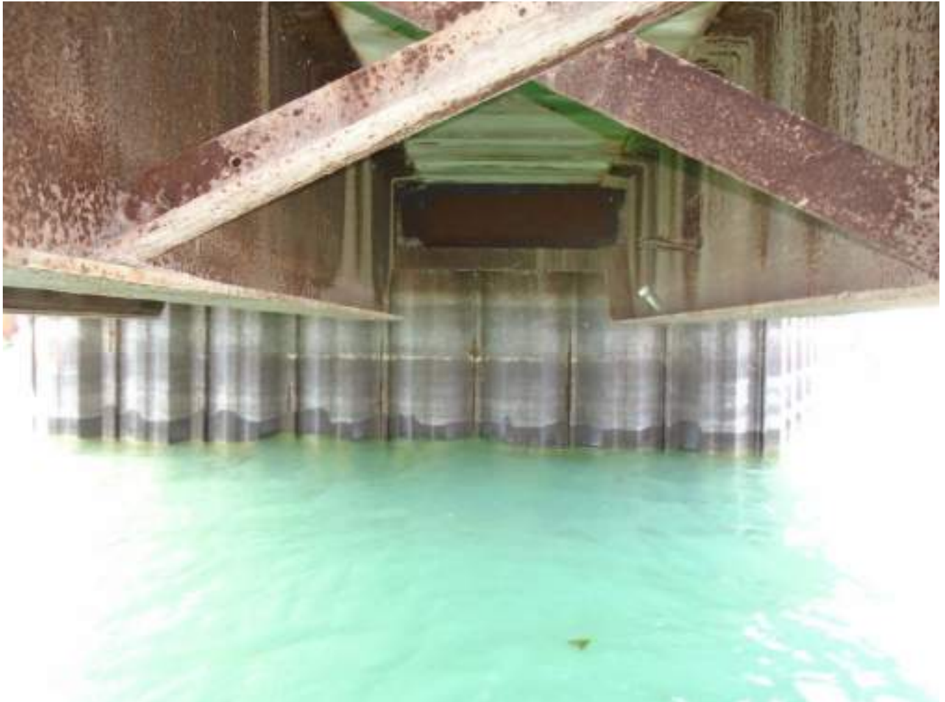
Looking West from East Abutment at Typical Cross Bracing Detail
