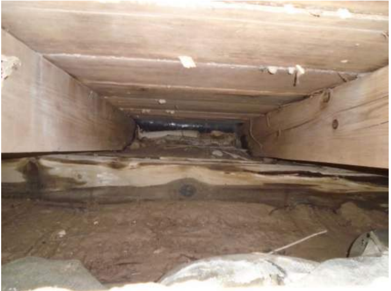
Looking north at north bearing beam
