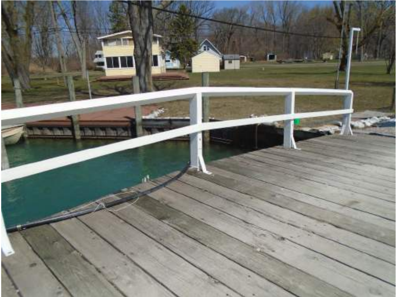
Looking NW at railing and deck
